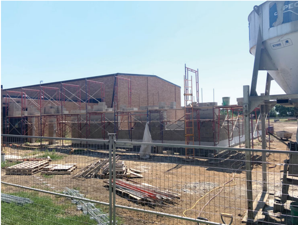
Construction is in full swing at SCC Elementary School in a photo taken on August 9 in Rockwell City. With most of the groundwork finished, the walls will rise following the start of the new school year. [Tyler Anderson/The Graphic-Advocate]
