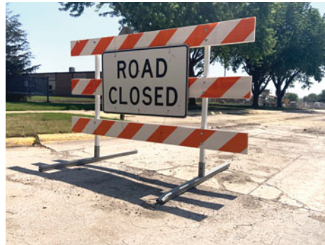
This “Road Closed” sign keeps incoming traffic at bay during the SCC Elementary expansion project, which was passed by the SCC Board of Directors in March. [Tyler Anderson/The Graphic-Advocate]
